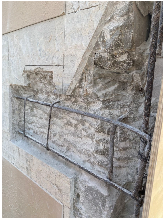
Picture 2: Concrete repair on the North stair tower
