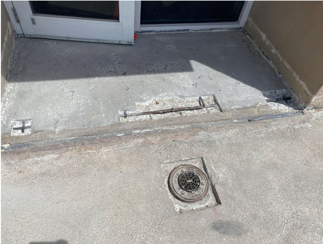
Picture 1: Concrete repairs at the entrance to the parking deck
